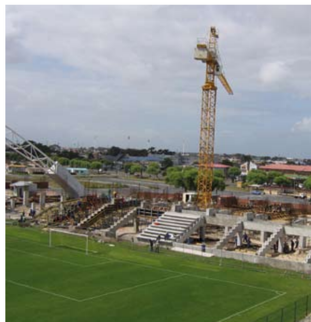
Athlone stadium under construction. Image: CSIR
