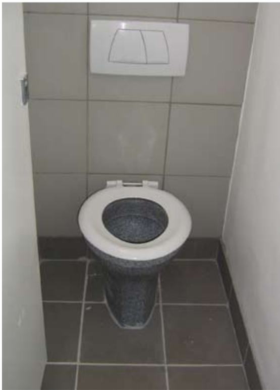
The new dual flush toilets. Image: CSIR
