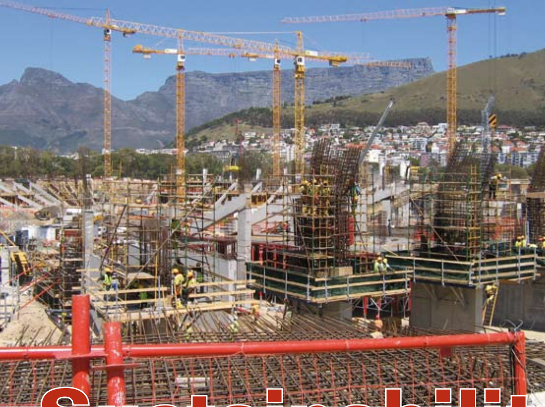
Green Point stadium, Cape Town, under construction. Image: CSIR
